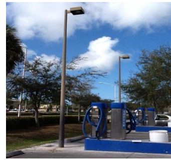
400 Watt Retrofit 93 Watt Car Wash Florida
